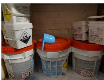
Incompatible chemicals stored on top of each other.
